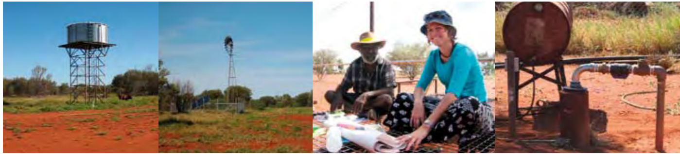
Water system infrastructure and community consultation at Mulga Bore.
