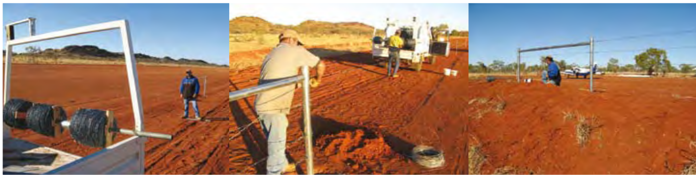
ITS team at work fencing the airstrip at Bonya.
