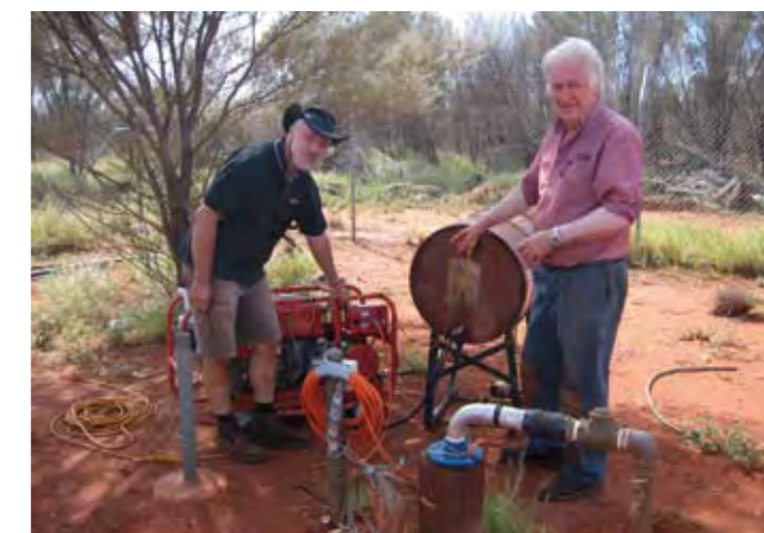
Water supply repairs at Mulga Bore.
