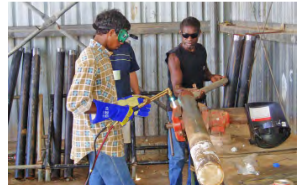
Welding training to construct bin stands, Wangkatjungka.
